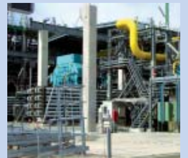
Primary Compressor in der LDPE-Anlage
